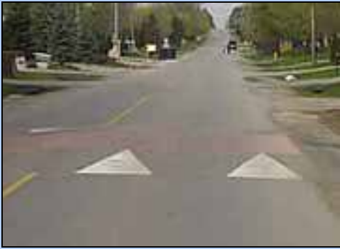
The raised cross-walk is an example of a traffic control technique that is achieved through design.
